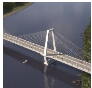
Ohio River Bridges East End Crossing Project
